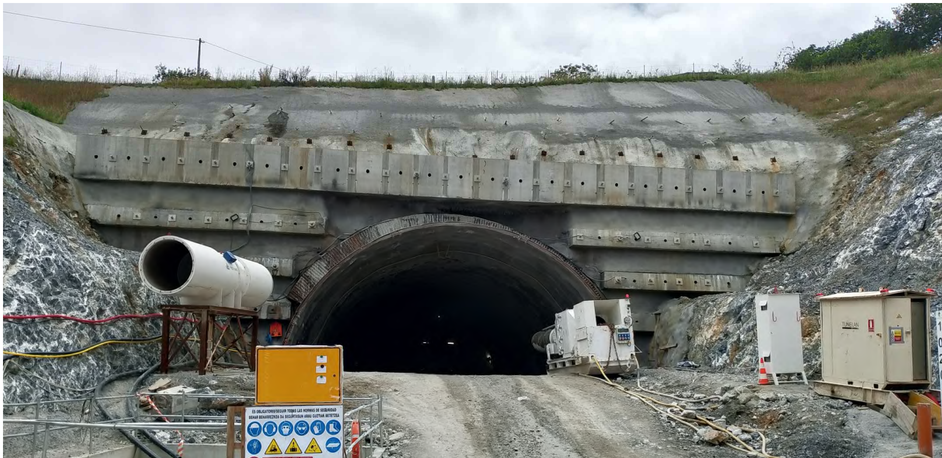
EMBOQUILLE TUNEL MARKINA
