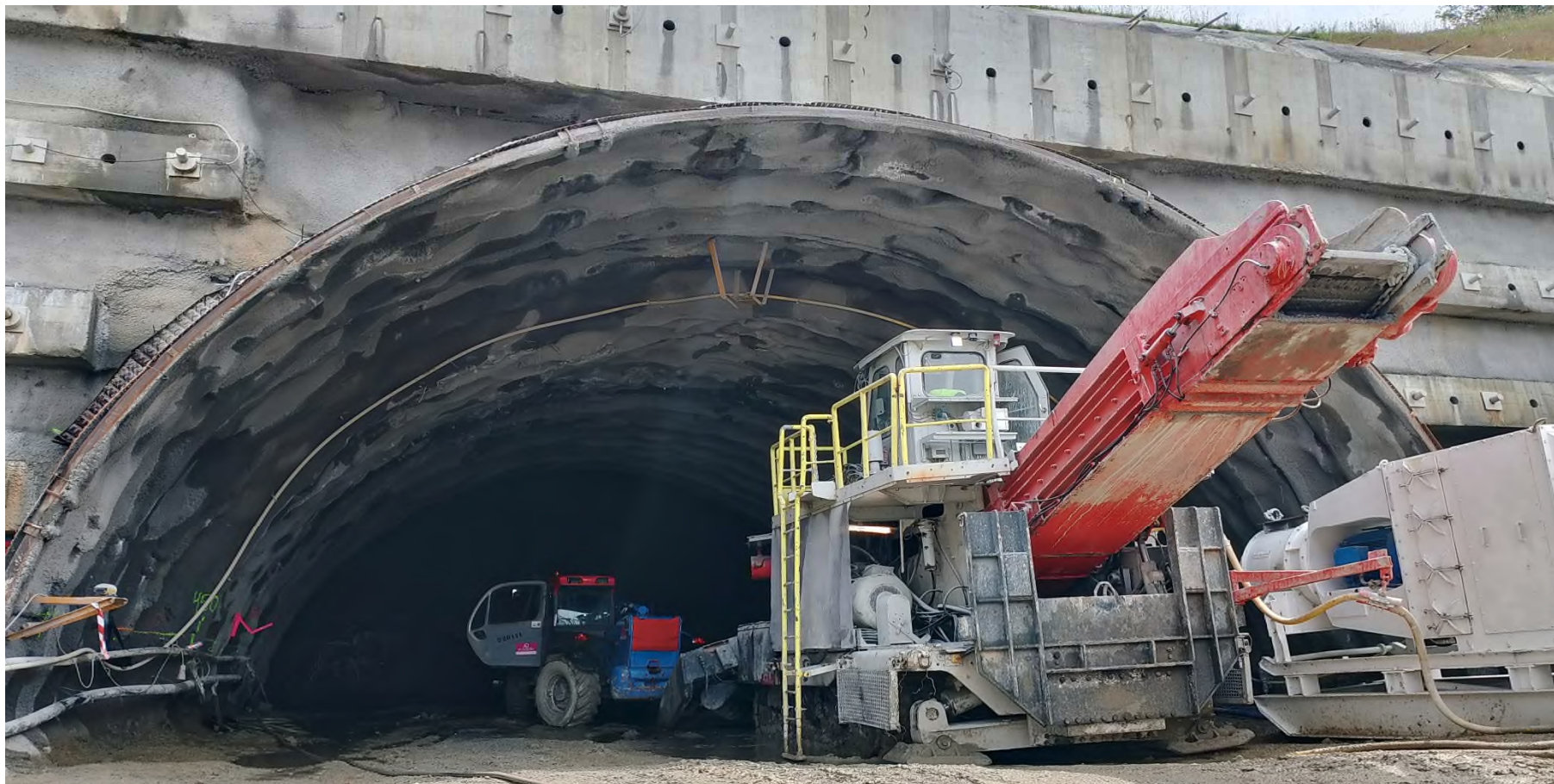
EMBOQUILLE TUNEL MARKINA
